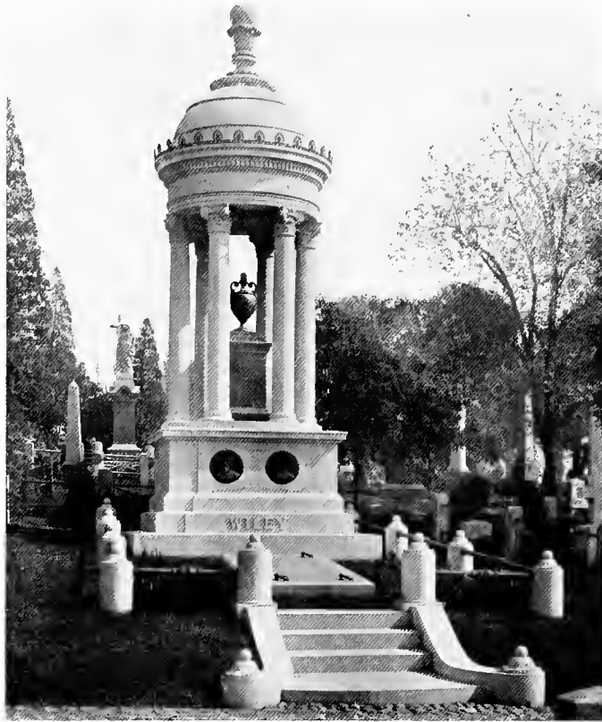
Number 8530. This magnificent canopy monument reflects the classical architecture of Rome in its artistic proportions and wealth of enrichment. A uniquely interesting feature is the removable slab immediately in front, disclosing an entrance to the underground vault having catacombs or niches for a number of interments. The main portions of the monument are of Barre Granite, on the pedestal of which are inserted finely executed, bronze medallion portraits. The bronze urn symbol surmounts a pedestal of dark Quincy Granite. The enclosure rail is also of bronze. The conception of the designers has been executed throughout with the greatest care. It is an excellent example of the high class of memorials we do. Erected in Greenwood Cemetery, Brooklyn, New York, for Estate of Annie Wiley.
